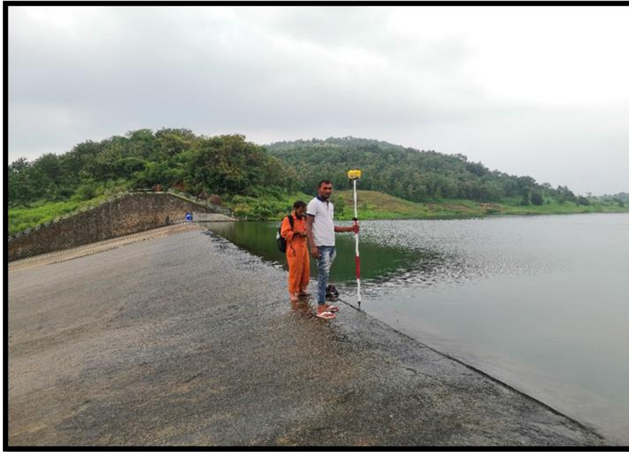
Top Level On Spillway
